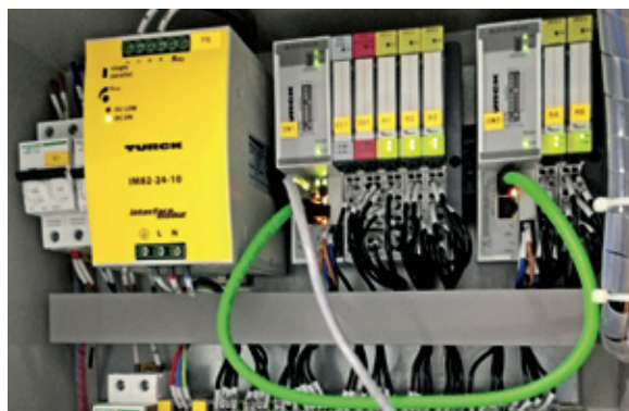
The BL20 RFID and I/O system from Turck ensures reliable communication with the PLC
